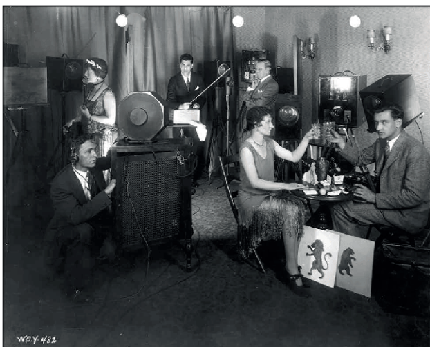
FIGURE 5. The right of the photo shows the “props” camera and the two people whose hands were reproduced. Props included revolvers, cigarettes, keys, rings, and so on. Above their hands is the “flying spot” projector, incorporating a light source, rotating disk, and lens. Behind each of the seated people are photo-cell boxes. In the center of the photo is a second similar camera setup.
